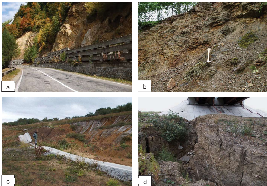
Figure 2. a) The Intramoesian Fault on the right bank of Lake Vidraru with cataclased augen gneisses and slope support works. b) The Intramoesian Fault in the northwestern Făgăraș Mountains, Moașa Sebeșului Valley, with cataclased micaschists. c) The cutting slope from Dealul Bucium with the destroyed drainage works and the broken protective nets. d) Deep ravine at the western head of the Aciliu Viaduct. Further explanations in text.
